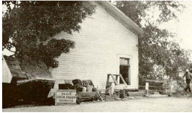
Bedford Corners Schoolhouse occupies the edge of the highway when it is moved from its foundation. – Mrs. Letha Baker
