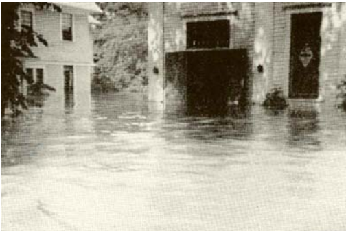
Water wasn't any higher at the Methodist Church, either. – D. H. Wing
