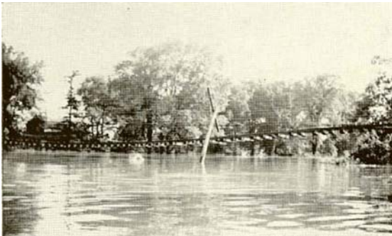
Pennsylvania Trestle at the Haskell where the bridge was completely wiped out. – Garden Inn
