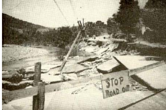
"Road Out" in front of Ed Johnson's home on Brooklyn Street. This was undermined by the Creek. – Thomas Pollock
